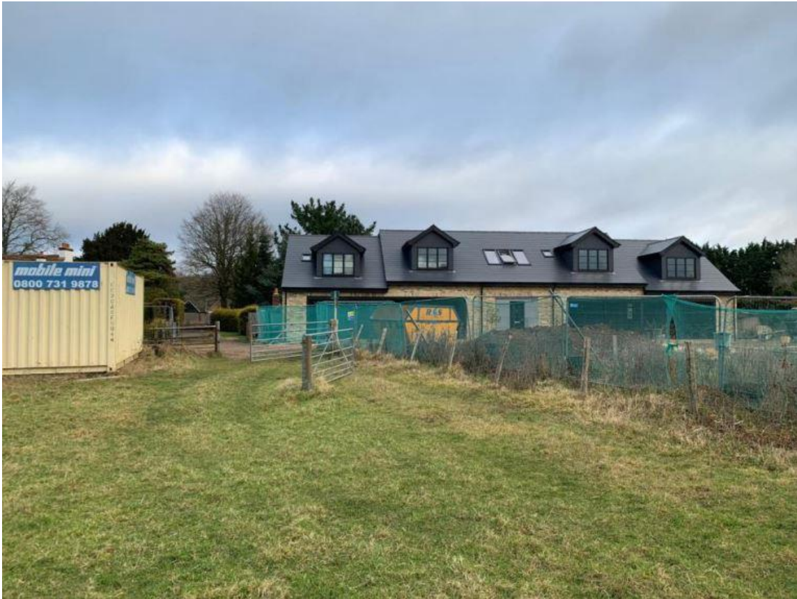
Photo 1 Existing rear elevation.
